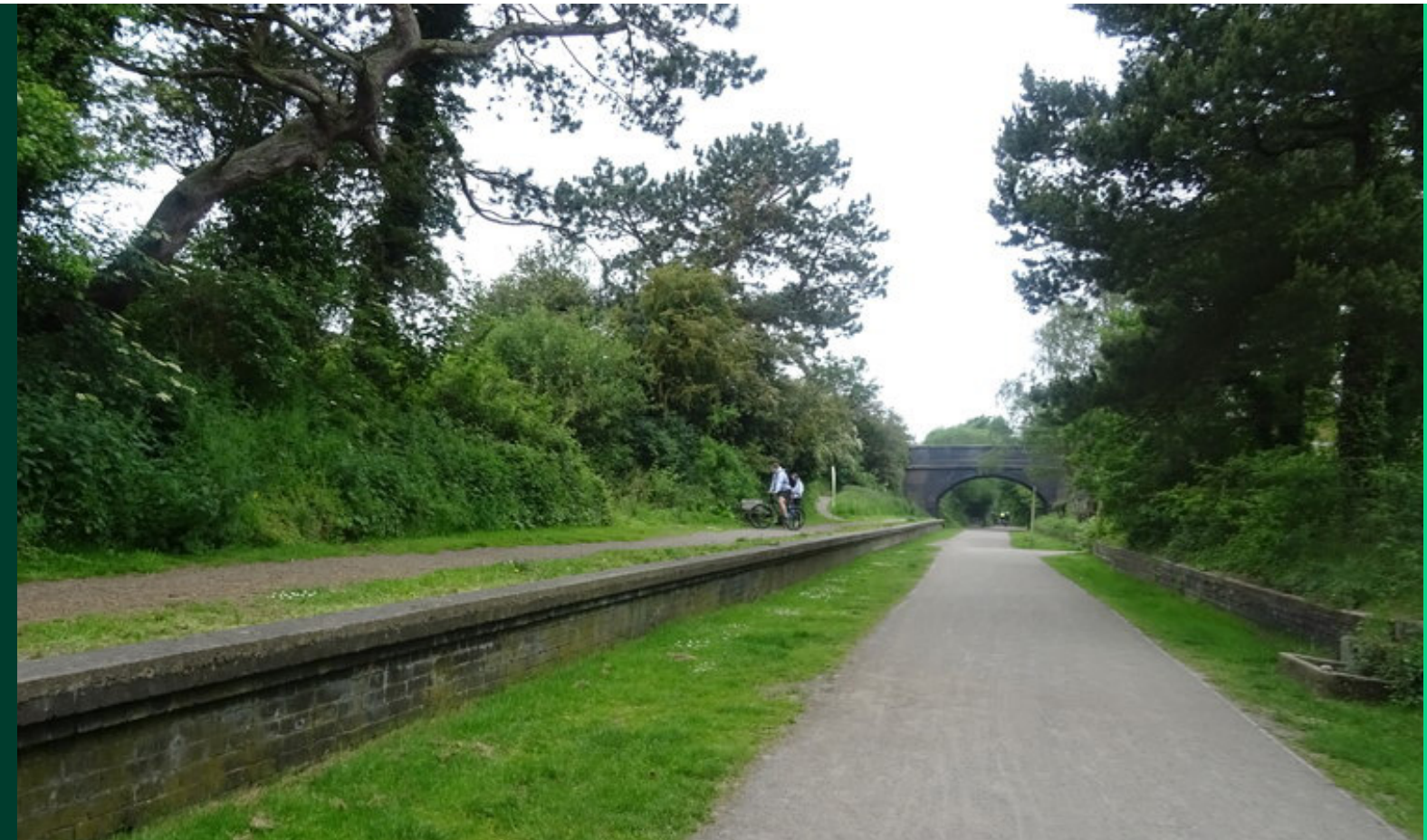
Segregated rural cycleway
