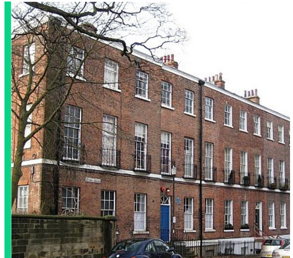
Brick Georgian facade
